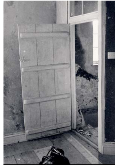
Attic door to back staircase
