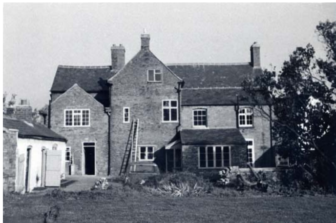
House Restoration Progressing 1967
