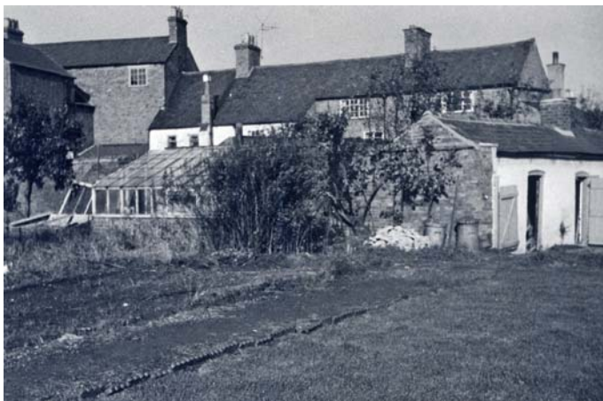
Garden improving 1967; greenhouse on the left and coal store on right
